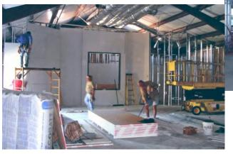
Above is the back wall of the auditorium in place. The two windows are for the media room on the left and the cry room on the right. At left the drywall is going up on the front of the auditorium. The
