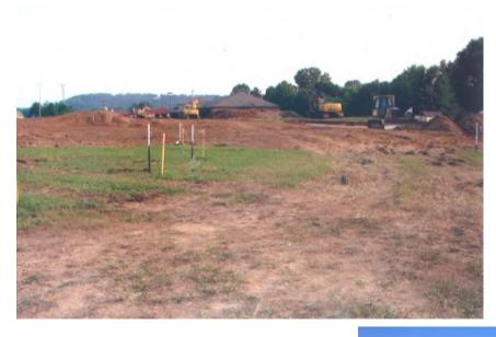
For several days the dirt crews worked. Finally all the dirt that would be under the slab was good dirt and it could be packed and leveled. Then the survey people came in and put stakes and string and flags, and more strings, until they were satisfied.
