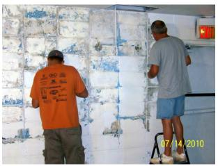
The photo on the left will be the rear of the auditorium. You can see a part of the small room that will be our "media room." After Carl painted the walls, which are concrete block, the paint bubbled and came off. There was mold all over one area. Time was spent scraping and wire brushing until we got it clean then Carl repainted.
